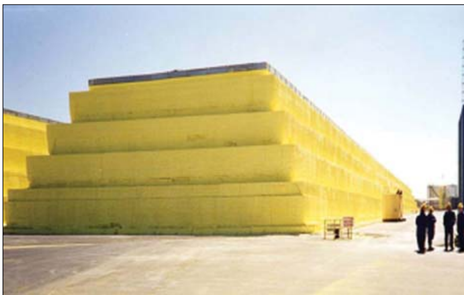
The tiered sulfur block resides on a sound base pad (Fig. 1).
