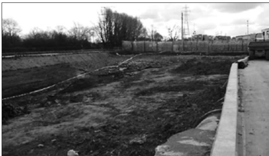
Four pipelines operated by UK's National Grid Gas PLC cross this location, the site of a future car park. Two of the pipelines operate at 32 bar, qualifying them as major accident hazard pipelines under UK Health and Safety Executive guidelines. Source: UK HSE (Fig. 1).
